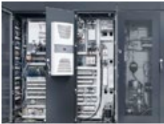
Climatic electric cabinet with easy access, isolated from heat sources.
